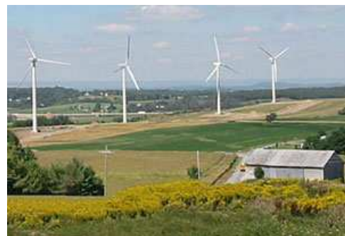
Exelon – Community Energy Wind Farm, Somerset County
