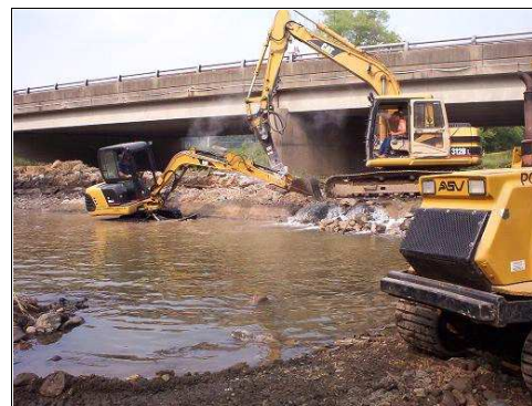
Removing Upper Dam on Wolf Creek
