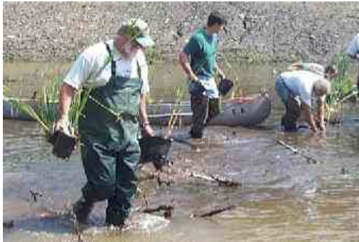
Ed helps plant “The Swamp” passive mine water treatment wetland.
