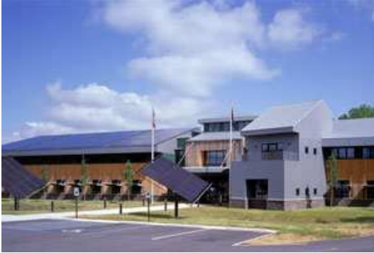
DEP Cambria Office with Solar Panels.
