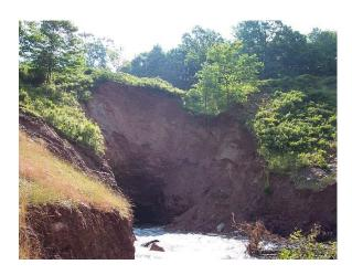
Flooding Blew Out the Audenreid Mine Discharge Tunnel Where It Attached to the Newly Dedicated Treatment System in Schuylkill County.
