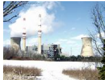
Montour Power Plant
