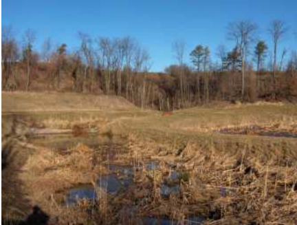
Boggs Run Treatment Facility Montour Run Watershed Allegheny County
