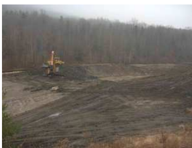
MaryD Reclamation Project, Schuylkill County
